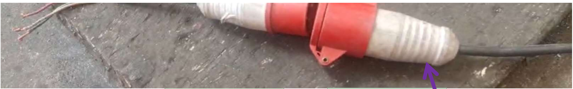
Left: 110V male connector (Plug) on end (插头)
